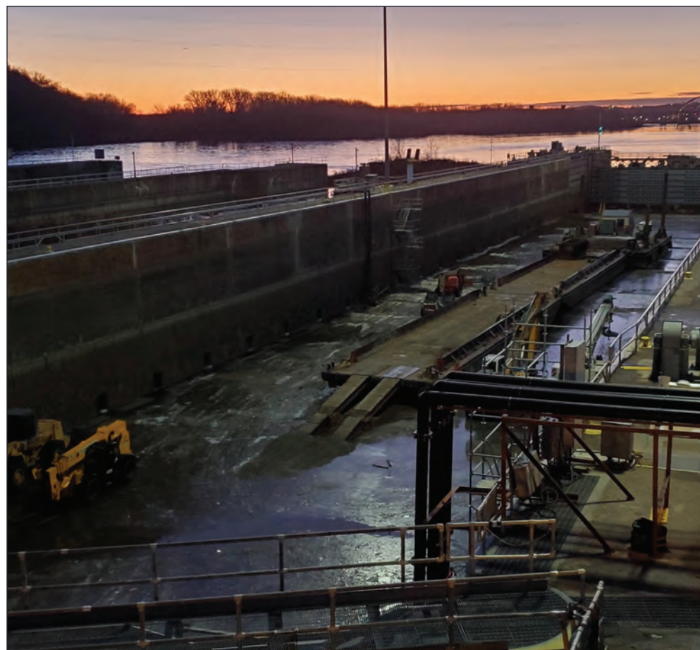
The dewatered lock chamber at Lock and Dam 2 in Hastings, Minnesota, Dec. 13, 2023. USACE St. Paul District photo by Patrick Moes
